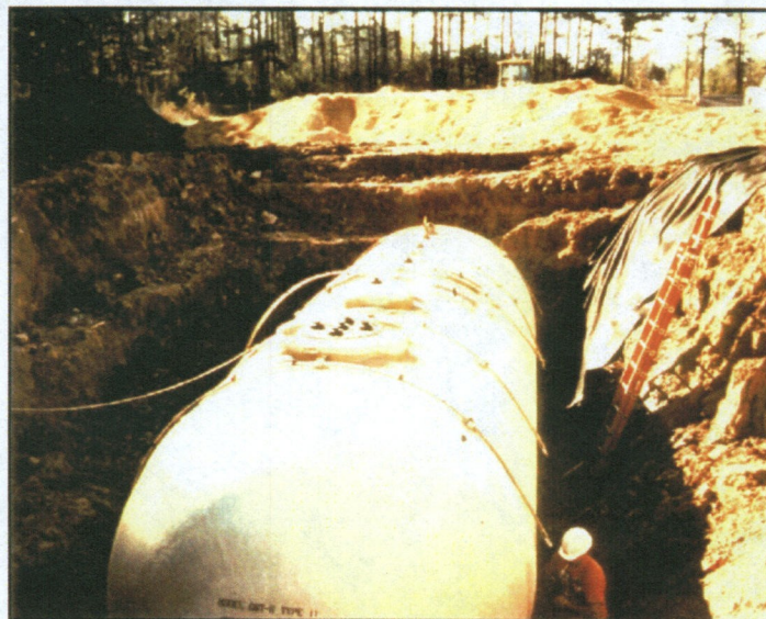
During an extensive and ongoing UST replacement program at Fort McClellan, an outdated steel tank was replaced with this double-wall, fiberglass fuel storage tank. The new 20,000-gallon capacity tank supports a major boiler plant on post and meets all regulator requirements under law.
